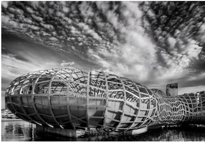
Bridge with a Difference
